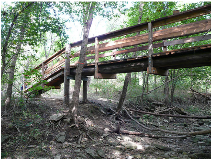
94 th Street Bridge
