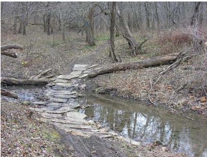
Jon Corkin – Mud Creek Armoring and Blue Trail Reroute
