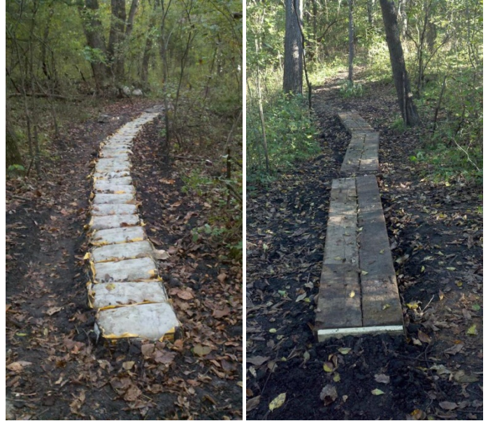
Quikrete & Railroad Tie Armoring
