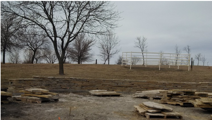
Groundwork and a retaining wall make way for a new open-sided shelter at West Point Equestrian Camp
