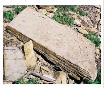
The quarried slices were then used to pave the trail as shown below. When the water rises and then recedes this armored trail tread will still be intact.
